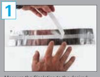
Measure the Sisalation to the desired length and peel back the doublesided tape backing
