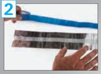
Measure the blue straping needed to go around the duct and back up to the hang point on the roof.
