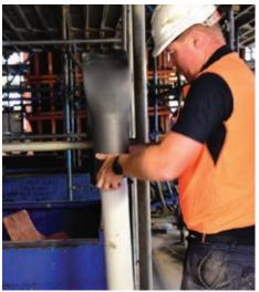
STEP 2: Cut to size and fit one end over the pipe and pull the sleeve onto the pipe.
